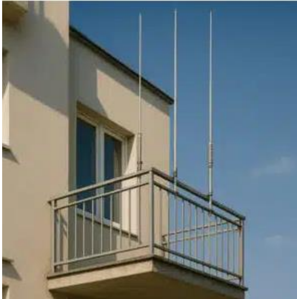
Vertical antennas mounted on balcony
