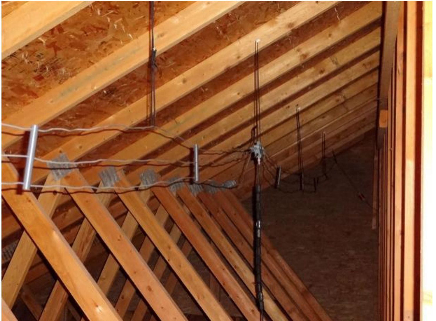
Fan Dipole with Coaxial Cable Feedline
